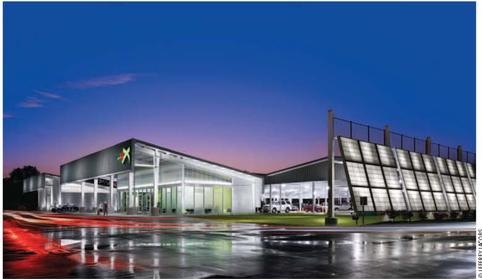
Here, 93 lights went into overdrive in this parking facility, replacing the existing lighting.
